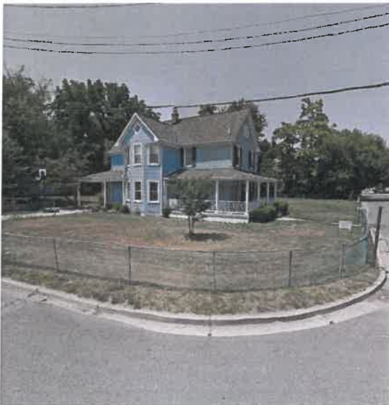
Existing fence at 8800 49 th Ave.
