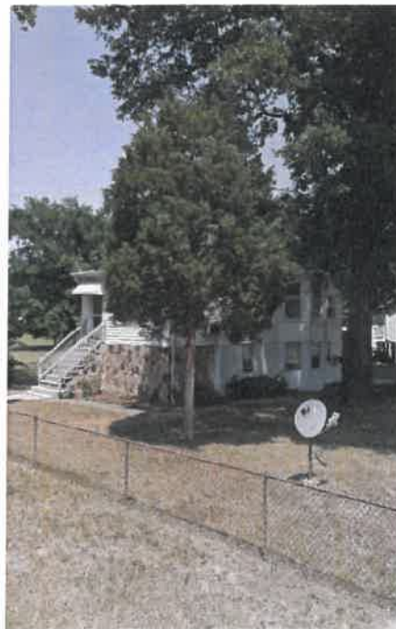
Existing fence at 8803 Rhode Island Ave.
